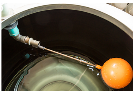
Level control float switch
